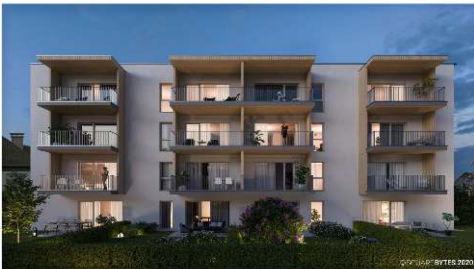
© Öko-Wohnbau/Novus Via in Villach
